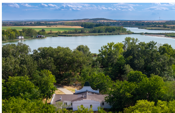
Forest lodge — aerial view
